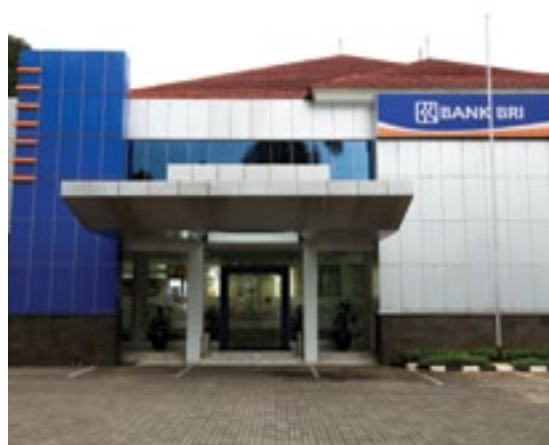
Branch Office Cut Mutia, Jakarta
