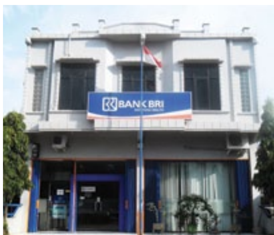
Sub-Branch Office Tugumulyo, Ogan Komeringlilir, South Sumatra
